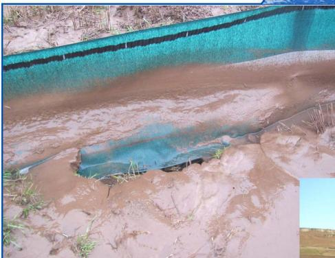
Ponding in Filter fence F led to cutting down to a stone drain
