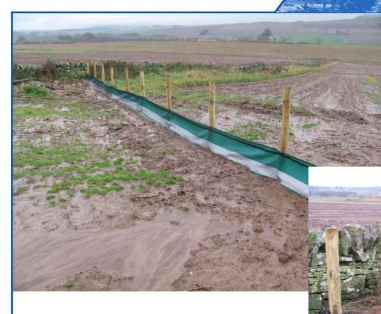
Filter fence A, showing diversion of flow and sediment into buffer strip which runs downslope for ca.200m).
