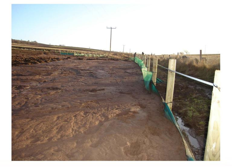
Note the natural filter mat forming on the coarse filter,
