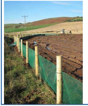
Terrastop<sup>™</sup> are designed to have catchment areas around 300 m<sup>2</sup> per m length of fence, which is restrictive for use in agricultural fields. therefore we have experimented with both Terrastop<sup>™</sup> and a much coarser, stiff **monofilament plastic netting** (pore space about 3mm), which we have used in combination with the finer netting.
