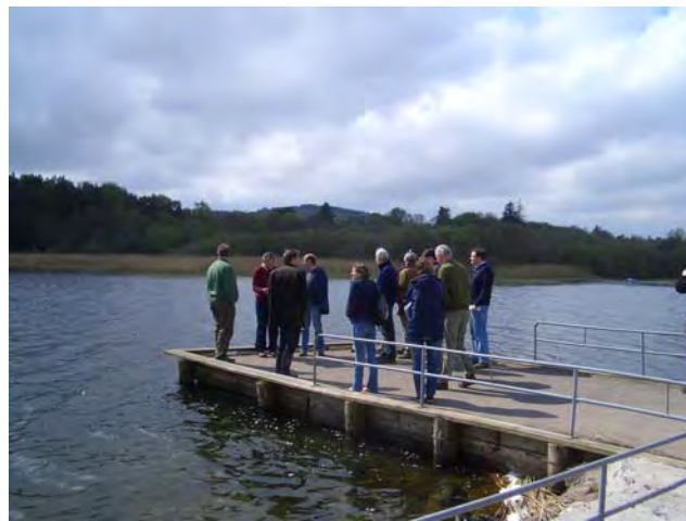
Figure 6c. Jetty at Rescobie Loch
